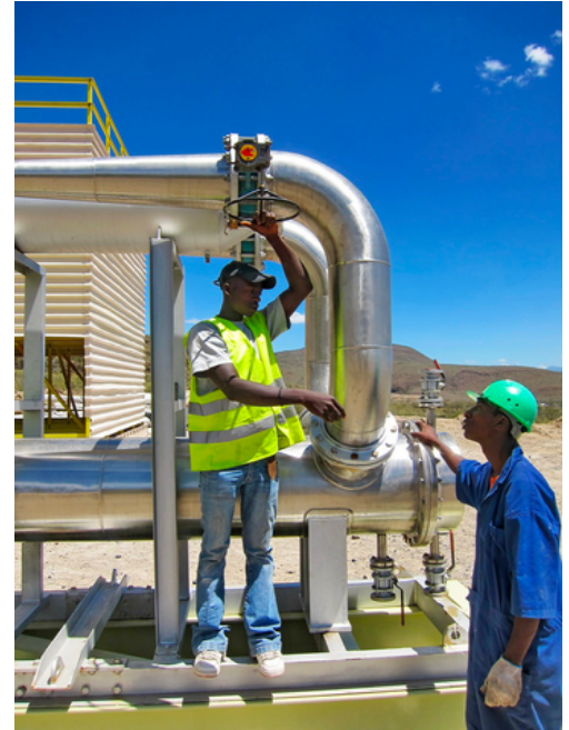
Workers at Olkaria Geothermal Power Plant, Kenya. Credit: Lydur Skulason, Flickr.
