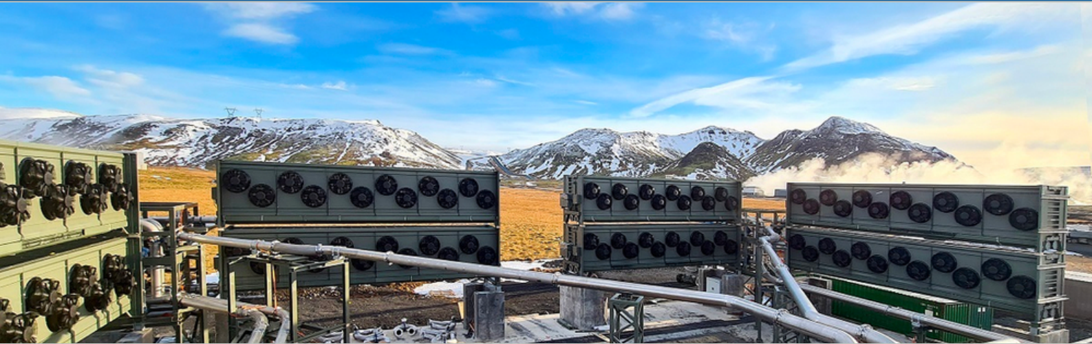
A Climeworks plant in Iceland can capture 4,000 tons of carbon annually. Business Wire/AP Photo
